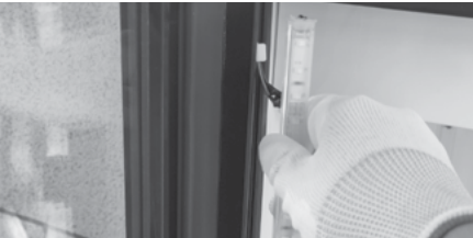
2 Take the light strip out of the slot.
