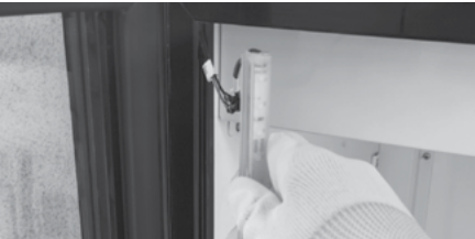
3 Disconnect the connecting terminals of the light strip and remove the light strip.
