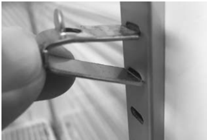
Securely insert shelf clips into pilasters
