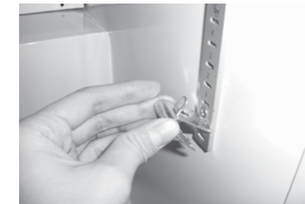
Securely insert shelf clips into pilasters.
